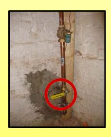
All fixtures except showers/tubs have a separate shut-off valve inside the house.
